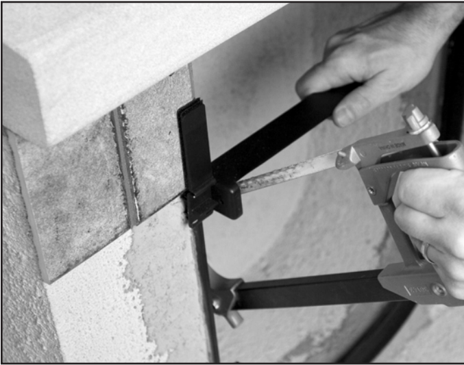
Diagram 27 - Cross Brace Removal
