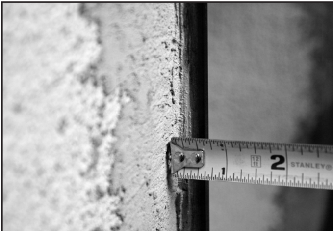
Diagram 26 - Plaster Ring - Troweled Mud
