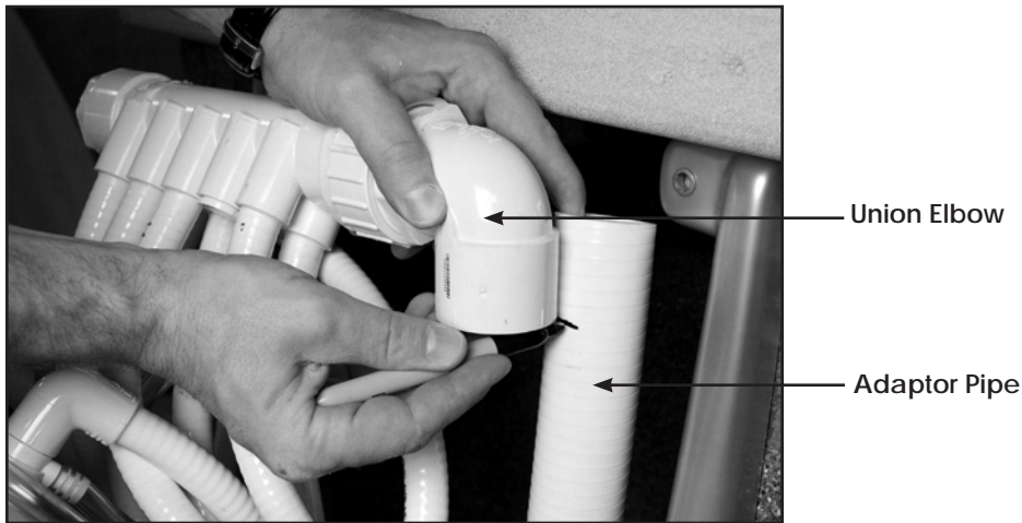
Diagram 41 - Marking Adaptor Pipe
