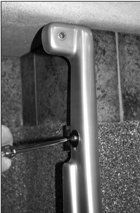
Diagram 35 - Secure Trim Ring to Plaster Ring
