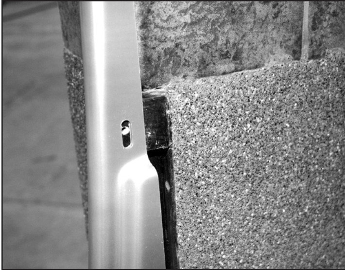
Diagram 34 - Line up Trim Ring with Plaster Ring
