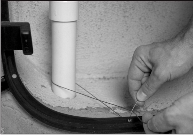
Diagram 25 - Secure Plaster Ring
