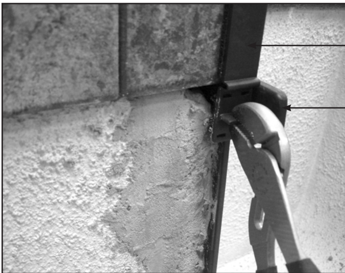
Diagram 28 - Upper Tab Removal
