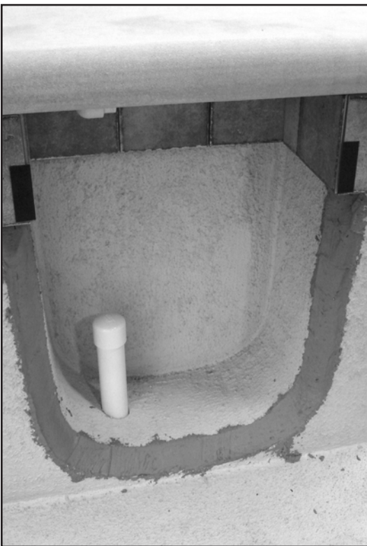
Diagram 23 - Mud Plaster Ring Notch
