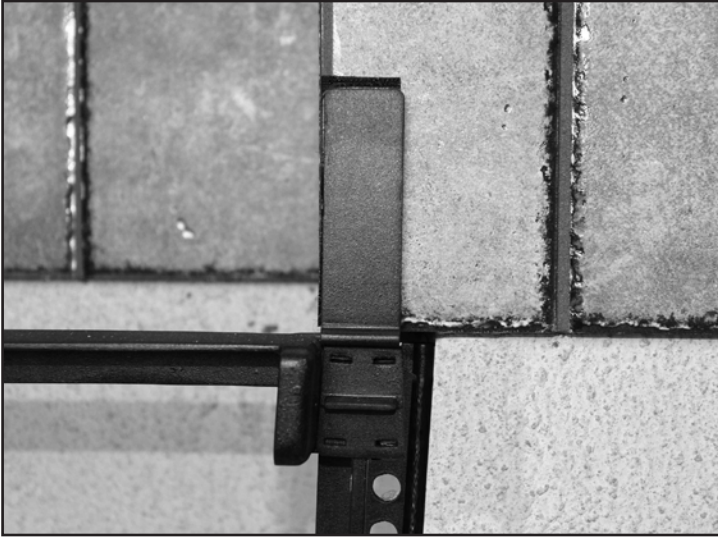
Diagram 21 - Velcro Plaster Ring to Tile
