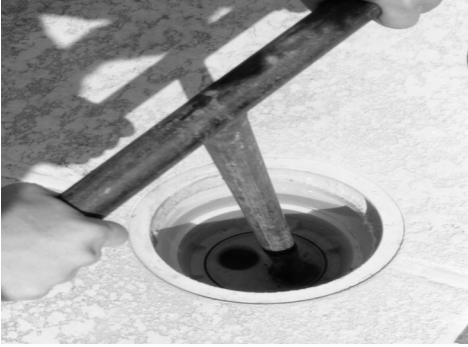
1. Remove all pressure test plugs.
