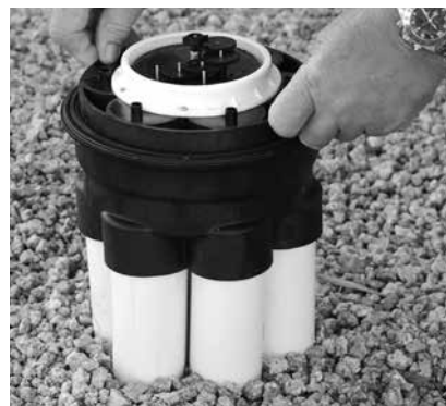
5. Turn module slightly until it sits in place lined up with guide pins
