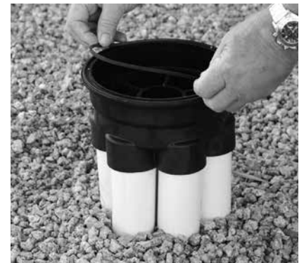
3. Clean and install base o-ring
