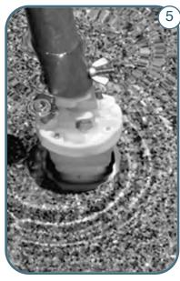
Press the top of the complete RetroJet nozzle onto the three prongs of the RetroJet installation tool. Guide the nozzle into the hole in the pool floor and then rotate clockwise 1/4 turn to lock in place. The nozzle will get tight as you turn it. When you feel a click, it has seated in the lock and is completely installed.
