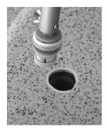
1. Use removal tool made for existing nozzle to remove one nozzle at a time by rotation 1/4 turn counter clockwise to unlock. The system is hydraulically balanced, so the same size nozzle needs to go back into the appropriate hole.
