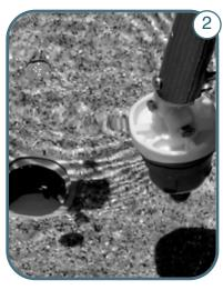
Use removal tool made for existing nozzle to remove one nozzle at a time by rotation 1/4 turn counter clockwise to unlock. The system is hydraulically balanced, so the same size nozzle needs to go back into the appropriate hole.
