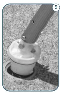
Press the top of the complete RetroJet nozzle onto the three prongs of the RetroJet installation tool. Guide the nozzle into the hole in the pool floor and then rotate clockwise 1/4 turn to lock in place.
