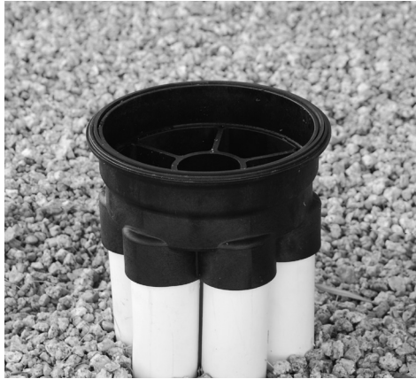
2. Remove clamp and dome
