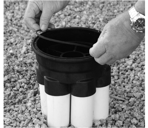
3. Clean and install base o-ring
