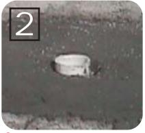
2. Cut off riser pipes flush with the concrete surface.
