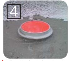
4. Glue the body into the pipe with HEAVY BODY PVC SOLVENT.
