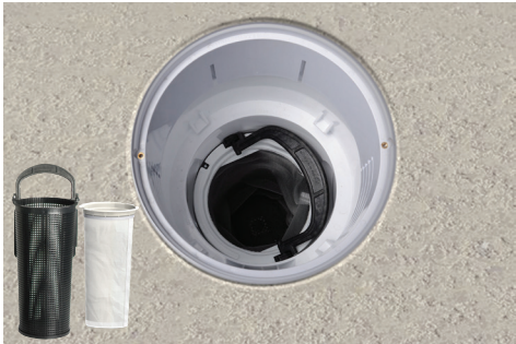
2. Install fine mesh bag and basket.
