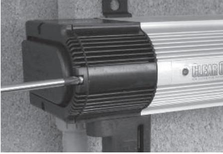
Turn the power off to filtration system pump at circuit breaker. Remove three screws in left end side cap labeled "electrical connections".
