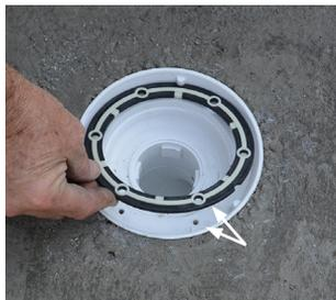
**2.** Place the seal ring within the body aligning the notches of the seal ring to the keys in the body. The seal ring is symmetrical and can be installed in either direction. Install the liner and make sure it is smoothed from the drain out past the area of the body you are working on.
