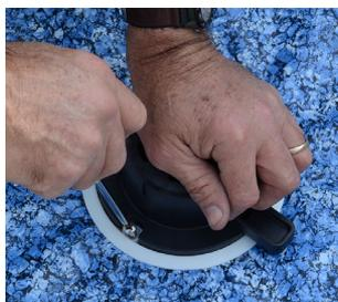
**5.** While firmly pressing down on tool with hand or knee, install two screws in opposite position evenly. Completely hand tighten screws. **DO NOT USE POWER TOOLS OR OVER TIGHTEN. MAX TORQUE (20 IN-LB.)**
