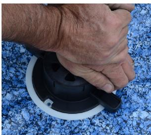
**4.** Once aligned, use the installation tool to uniformly seat the clamp ring to the body. Align cutout in tool for access to screw holes.
