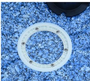
**7.** Be sure each screw head is below the clamp ring gauge. **DO NOT OVER TIGHTEN.**
