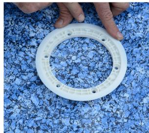
**3.** Align the clamp ring over the body. There are 3 bumps on the body that corresponds with notches in the clamp ring (see step 2).
