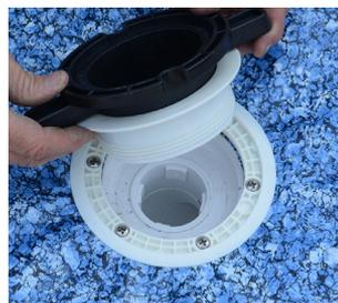
**9.** Using the other side of the installation tool, tighten the threaded trim ring to the body.
