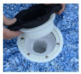
Using the other side of the installation tool, tighten the threaded trim ring to the body.
