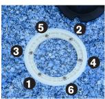
Rotate the installation tool, press down again and install remaining screws in the order shown above.
