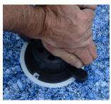
4. Once aligned, use the installation tool to uniformly seat the clamp ring to the body. Align cutout in tool for access to screw holes.
