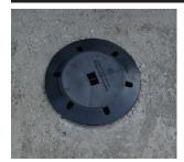
1. Before pouring concrete around the Vanish™ body be sure the cap is on the body. Pour concrete in a 12"x12"x6" deep area and trowel smooth with the flange on the body and the finish level of the vermiculite. Be careful not to get concrete in the screw holes.
