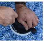
While firmly pressing down on tool with hand or knee, install two screws in opposite position evenly. Completely hand tighten screws. DO NOT USE POWER TOOLS OR OVER TIGHTEN. MAX TORQUE (20 IN-LB.)
