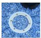
Be sure each screw head is below the clamp ring gauge.DO NOT OVER TIGHTEN.
