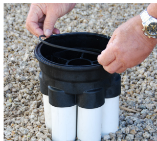
3. Clean and install base o-ring
