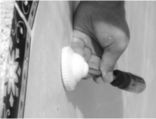
Proper Positioning Of Down Jet Eyeball
